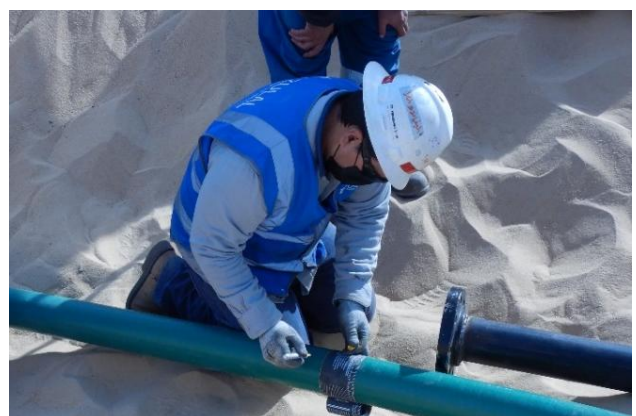
Photographs, Dec-2021: Completed in just one day, the deployment of 1038 meters Fiberspar Spoolable 4" FSLP 750 series LinePipe for Well No. M-31 flow line at Zaggut Station of Waha Oil Company.
