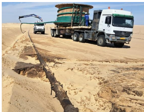
Photographs, Oct-2024: At Waha Oil Company's well # A-134, Fiberspar 6" 750X RTP pipe is being installed as flowline 1.3km length, beside a corroded Carbon Steel CS pipeline leaking crude oil.
