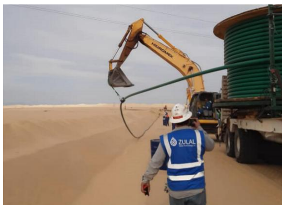
Photographs, Dec-2021: Completed in just one day, the deployment of 1038 meters Fiberspar Spoolable 4" FSLP 750 series LinePipe for Well No. M-31 flow line at Zaggut Station of Waha Oil Company.
