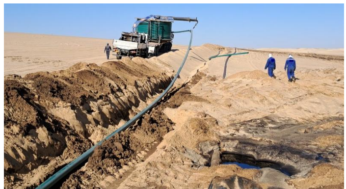
Photographs, Oct-2024: At Waha Oil Company's well # A-134, Fiberspar 6" 750X RTP pipe is being installed as flowline 1.3km length, beside a corroded Carbon Steel CS pipeline leaking crude oil.
